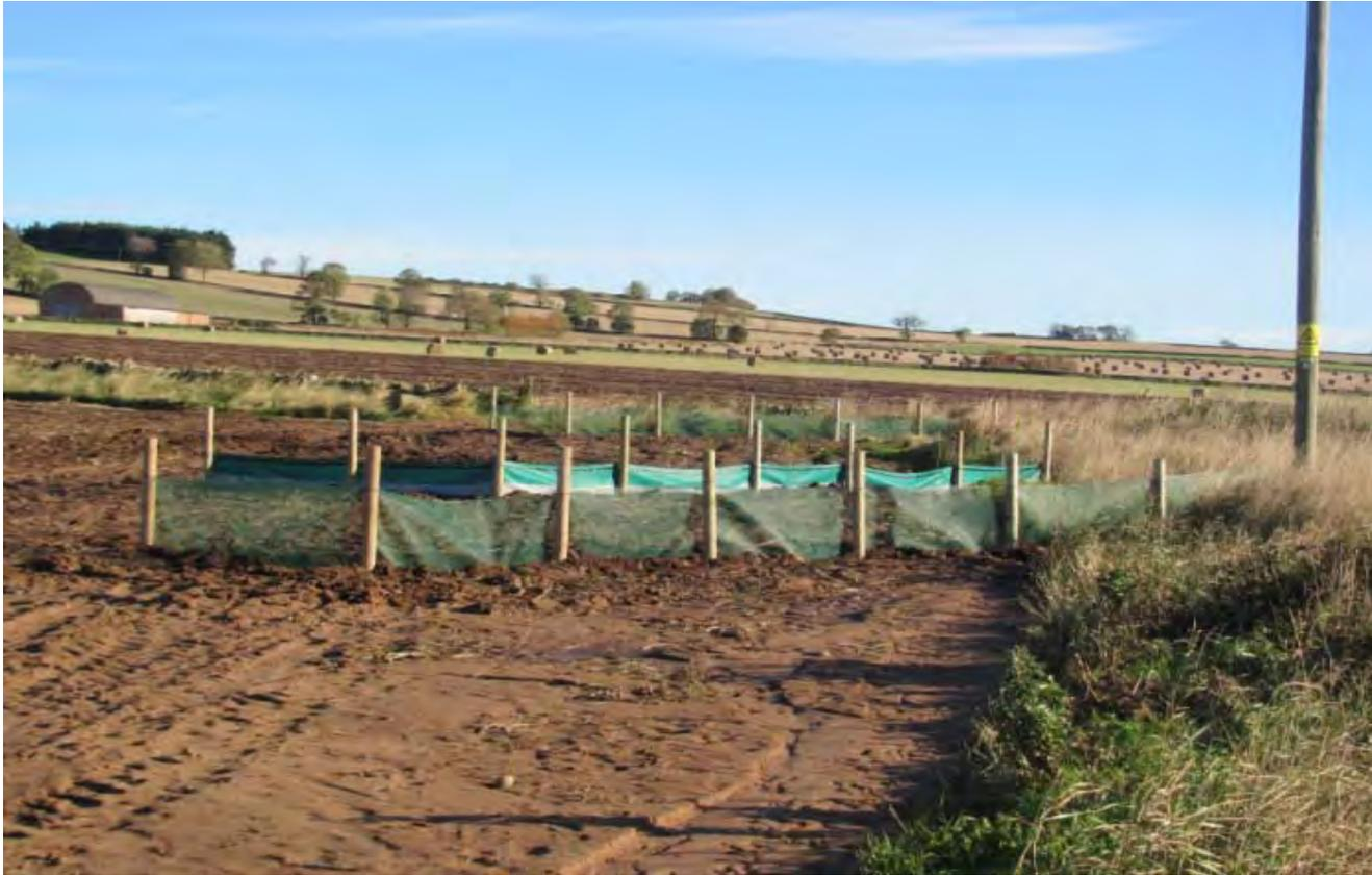
Filter fences B (furthest away, coarse filter),
