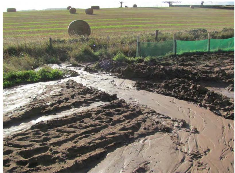
**Terrastop™ Premium** is a special, high quality, permeable, technical filter fabric that can be installed as an entrenched vertical entrapment fence, and is designed to intercept and detain run-off, trapping harmful silt through settlement and filtration before it leaves the site.
