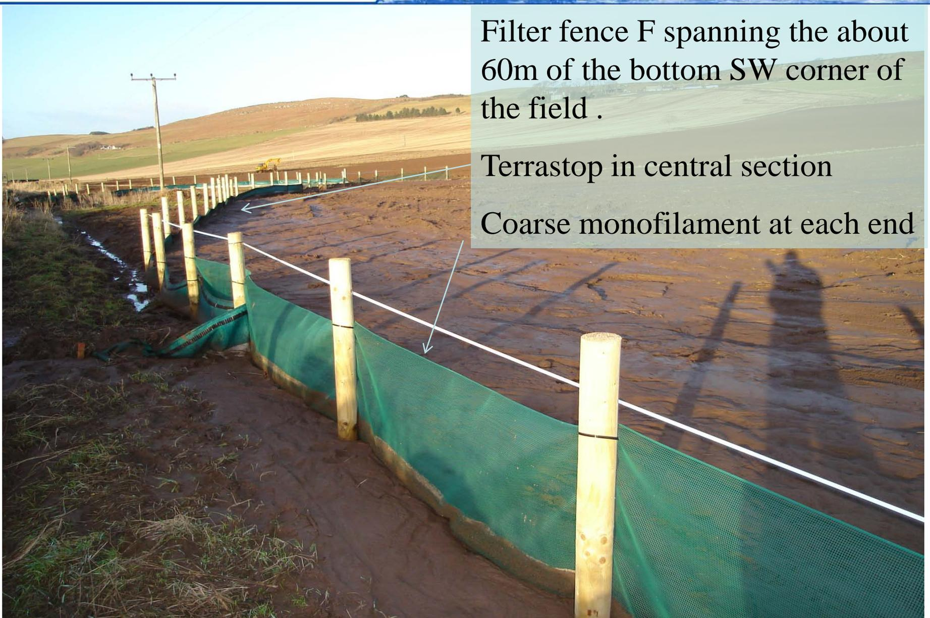
Filter fence F spanning the about 60m of the bottom SW corner of the field .
