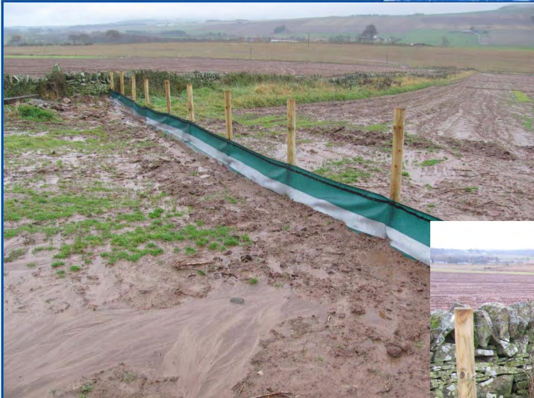
Filter fence A, showing diversion of flow and sediment into buffer strip which runs downslope for ca.200m) .
