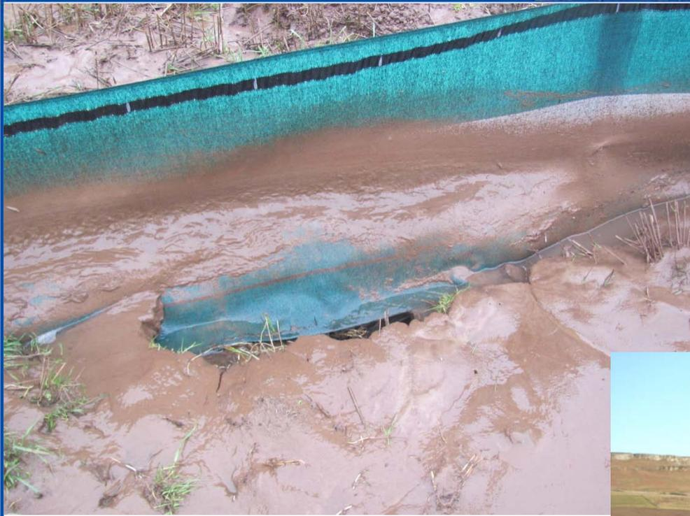
Ponding in Filter fence F led to cutting down to a stone drain
