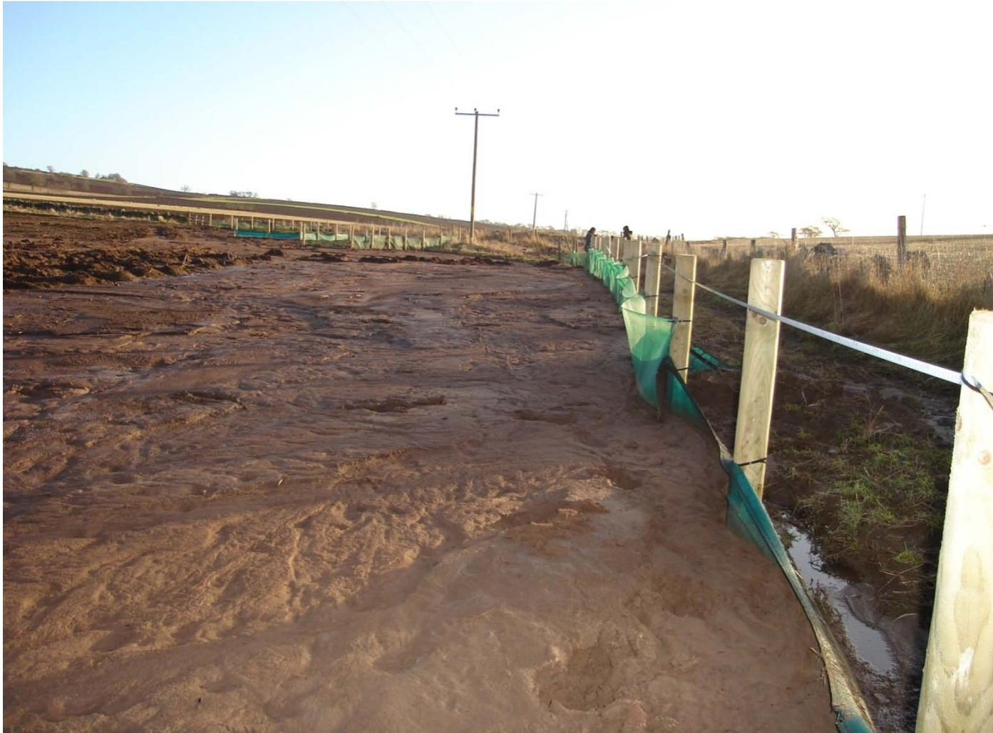
Note the natural filter mat forming on the coarse filter, which helps the water to spread along the contour and deposit its sediment load
