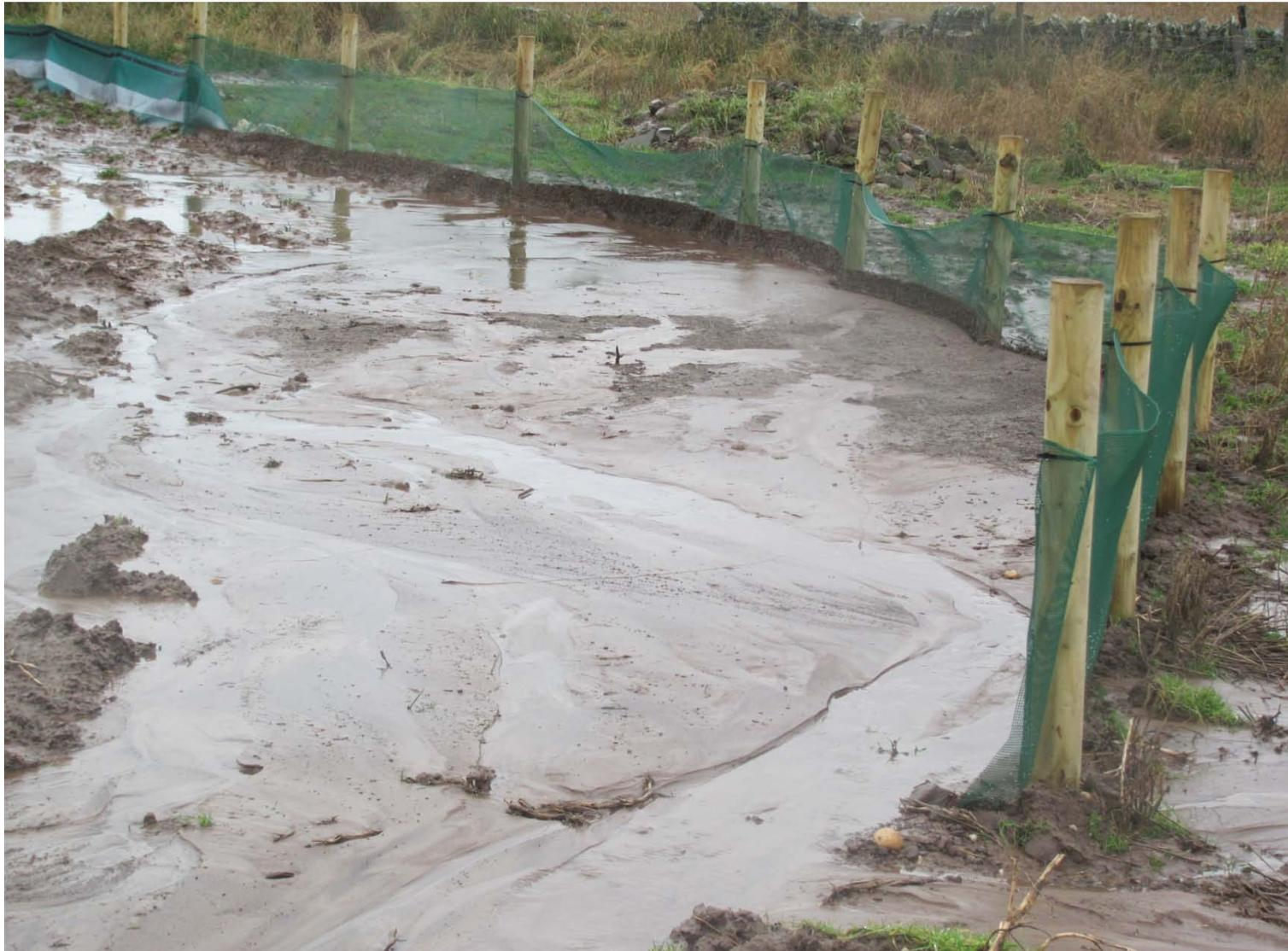
About 40 tonnes of sediment had accumulated in filter E by 1 Feb
