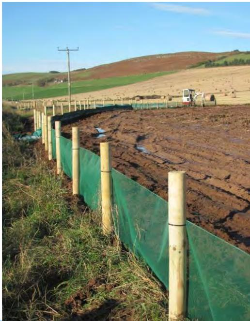
Terrastop™ are designed to have catchment areas around 300 m<sup>2</sup> per m length of fence, which is restrictive for use in agricultural fields. therefore we have experimented with both Terrastop™ and a much coarser, stiff **monofilament plastic netting** (pore space about 3mm), which we have used in combination with the finer netting.
